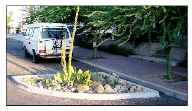
Old style curb extension built by the City as part of the Stone Avenue improvements does not have curb openings to allow water to flow into the landscaped basin. Avenue.
