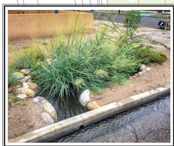
Curb core hole directs street runoff to street-side basin. This basin harvests over 4,500 gallons annually. Photo: Brad Lancaster
